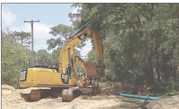
Woodside Heights sewer line construction
